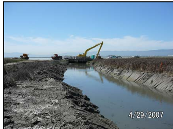
Figure 3-3: Pond A14 post construction of channel
